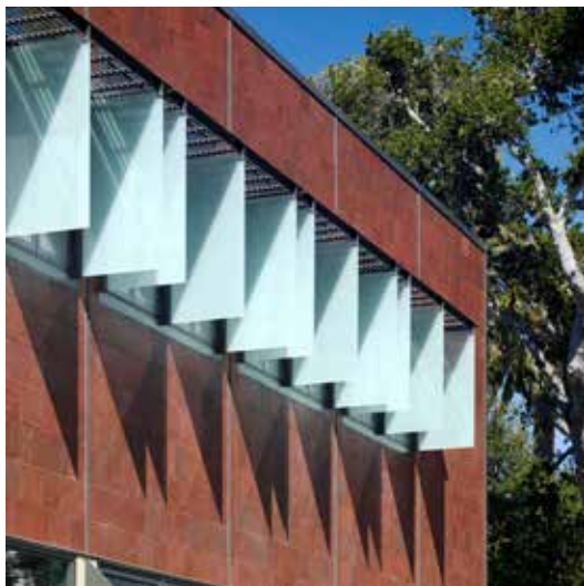
South exposures should be articulated to control solar gain (upper). East and west-facing windows may require vertical solar shading (lower).
