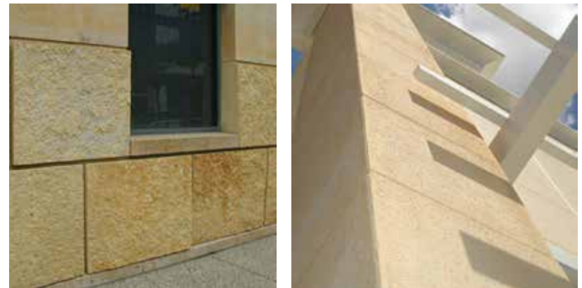
Use of natural stone enhances building color and texture (above left and right).
