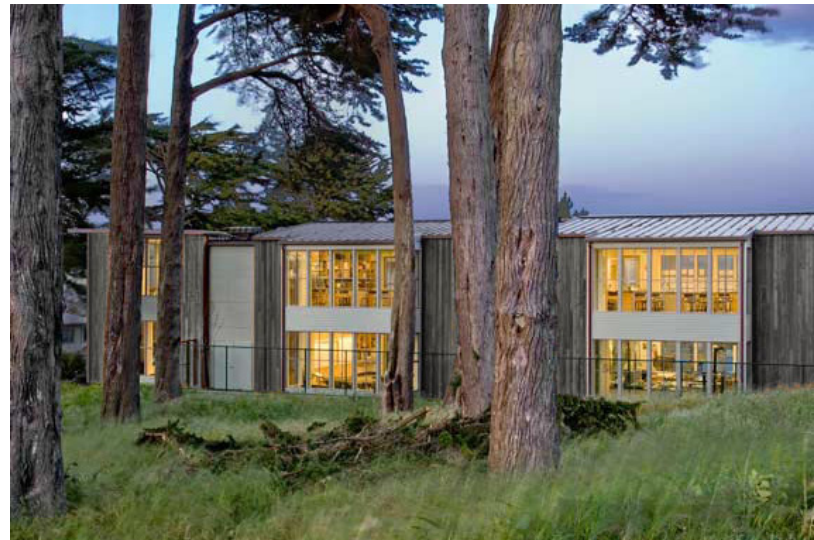
Building forms providing interaction with the environment (upper); building siting responsive to landform and landscape (lower).
