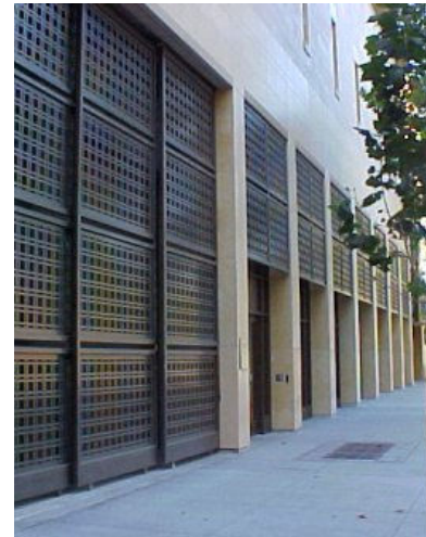
Design service docks and loading areas in keeping with building envelope (left). Screen service areas from view and isolate to mitigate noise with physical barriers including landscape (right).
