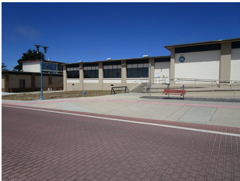
Figure 2. Main (west) elevation, looking northeast (IMG_0654)
