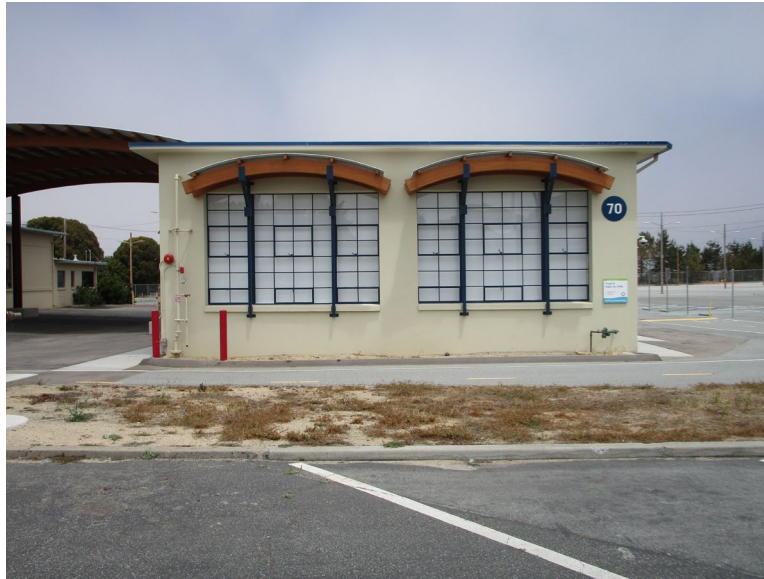
Figure 1. Main (south) elevation, looking north (IMG_0335)
