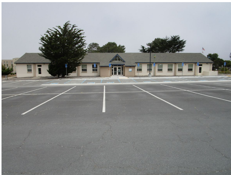
Figure 1. Main (south) elevation, looking north (IMG_0302)
