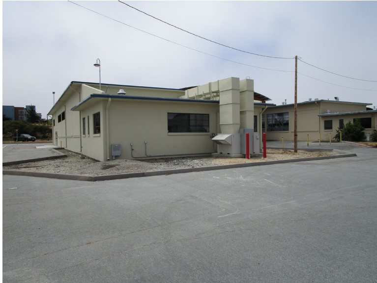
Figure 2. North (right) and east (left) elevations, looking southwest (IMG_0348)
