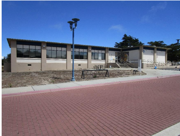
Figure 23. Building 44, Pacific Hall, View facing east at the west elevation (IMG_0602).
