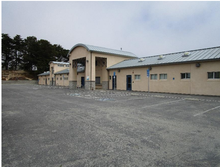
Figure 24. Building 902, Freeman Stadium, View facing northeast at the west elevation (IMG_0431).
