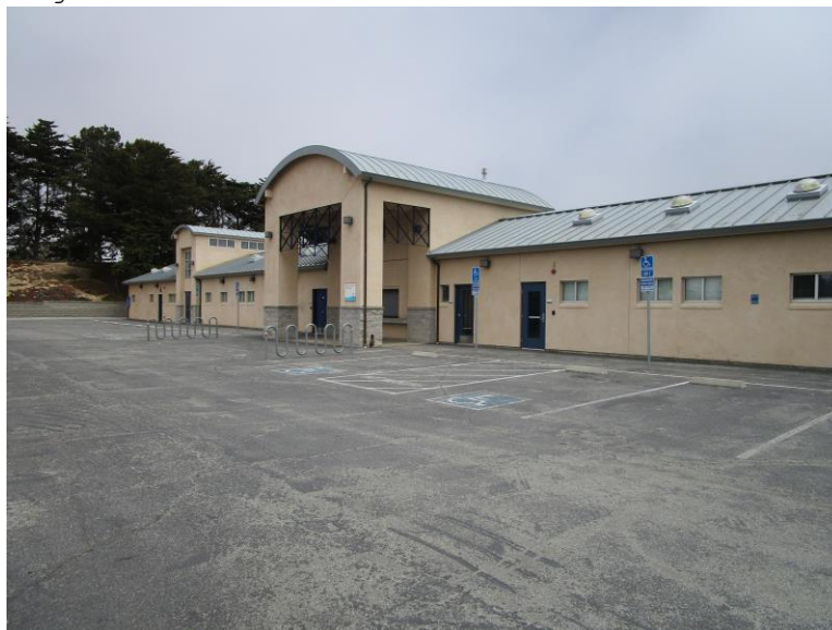
Figure 1. Main (west) elevation, looking northeast (IMG_0431)
