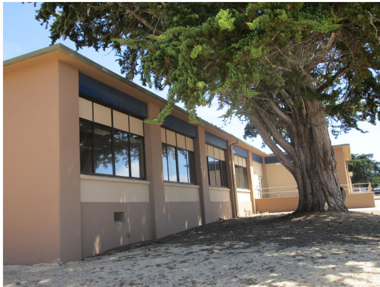
Figure 1. Main (west) elevation, looking southeast (IMG_0644)
