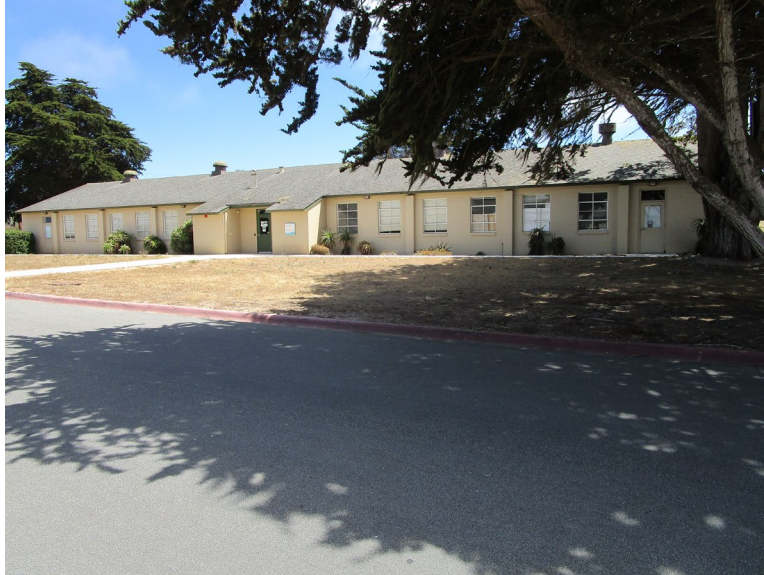
Figure 1. Main (north) elevation, looking southeast (IMG_0566)
