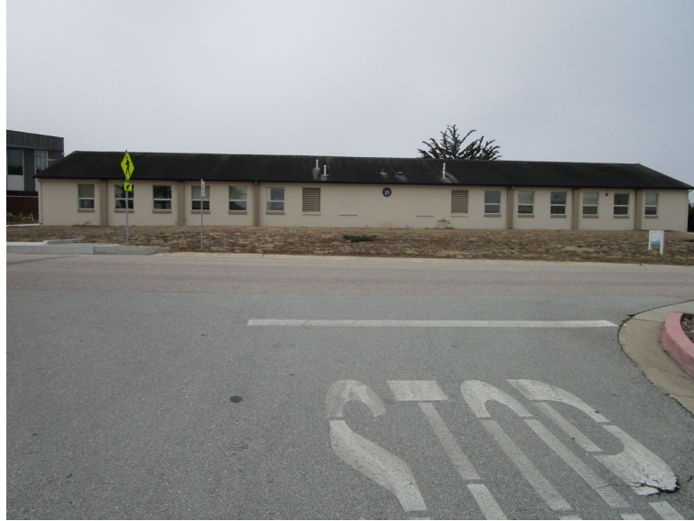
Figure 2. North elevation, looking south (IMG_0314)
