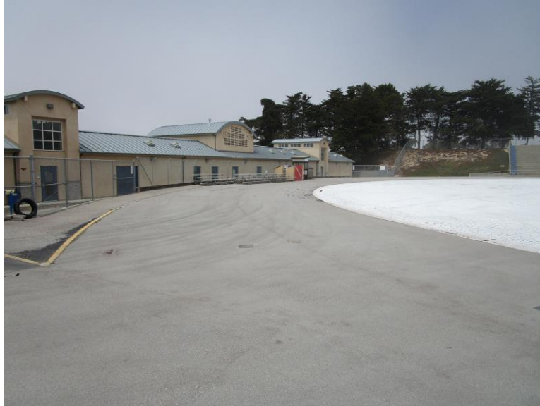
Figure 6. Track detail, looking northwest, Field House in background (IMG_0437)
