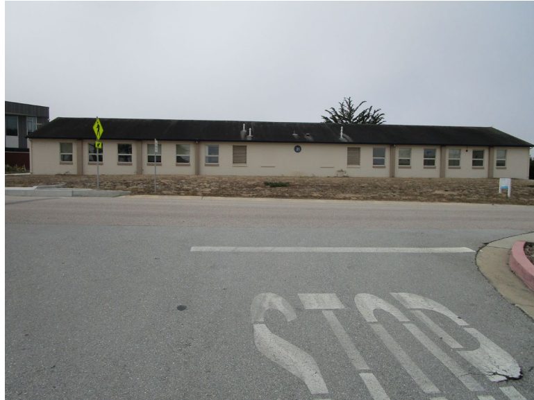
Figure 2. North elevation, looking south (IMG_0314)
