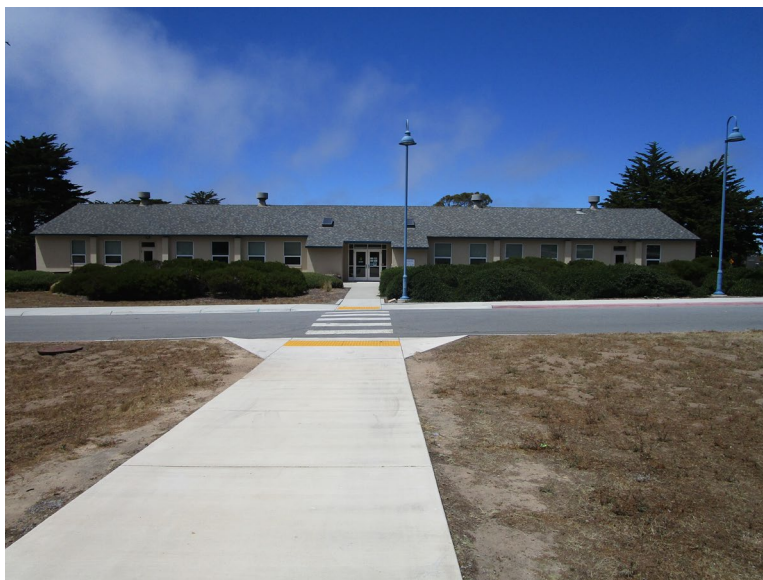
Figure 1. Main (south) elevation, looking north (IMG_0581)
