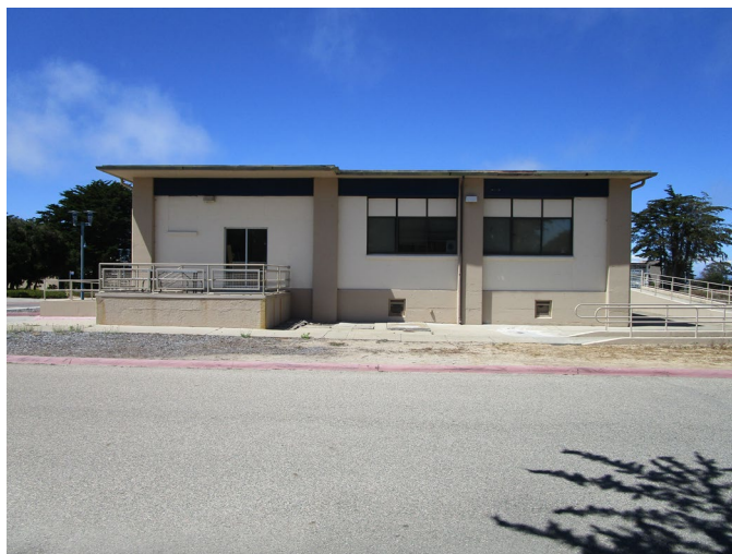
Figure 2. South elevation, looking north (IMG_0621)
