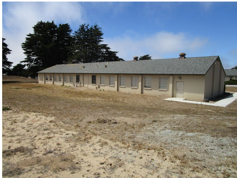
Figure 2. South elevation, looking northwest (IMG_0576)
