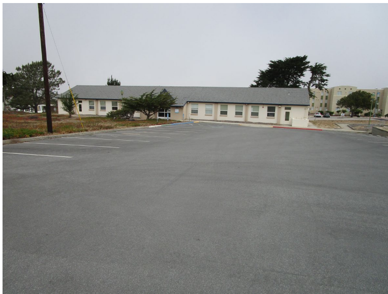
Figure 1. Main (south) elevation, looking north (IMG_0292)
